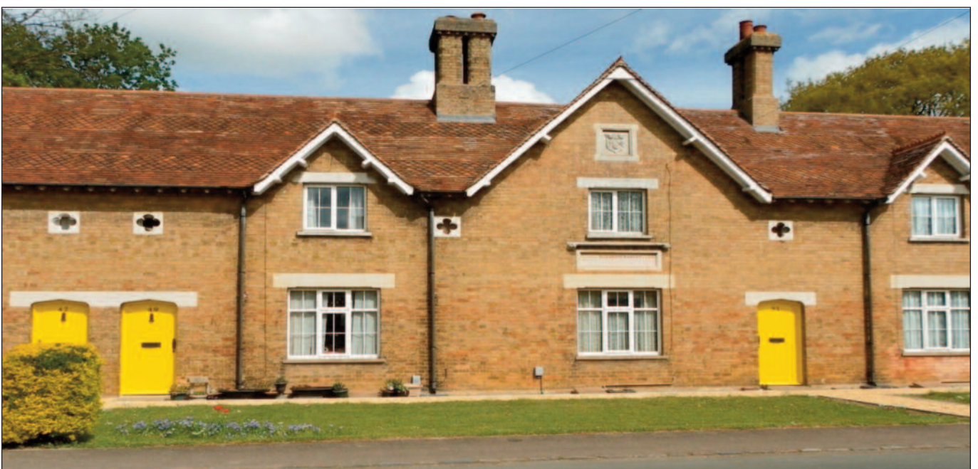
Elizabeth Harvey Alms Houses Upper Caldecote
