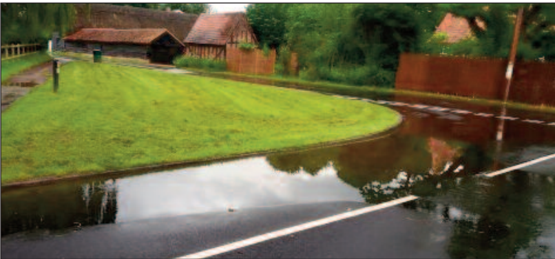
Blocked gully in Ashby Drive
